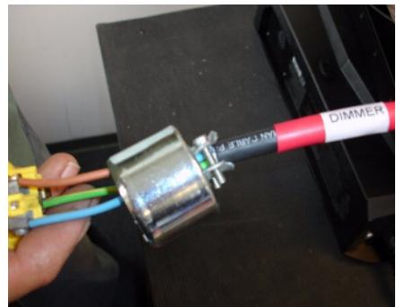
**2** Install the attachment plug to the dimmer power cord.
